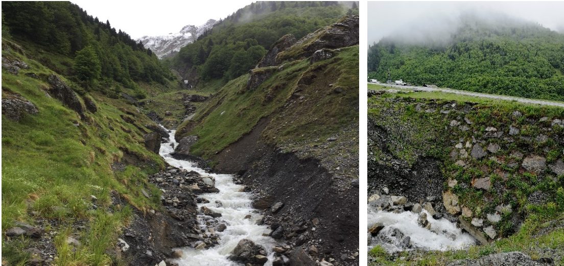
Figure 4.10 The torrent at Socques. Erosion in easily erodible deposits (left), and the partly blocked culvert (right).
