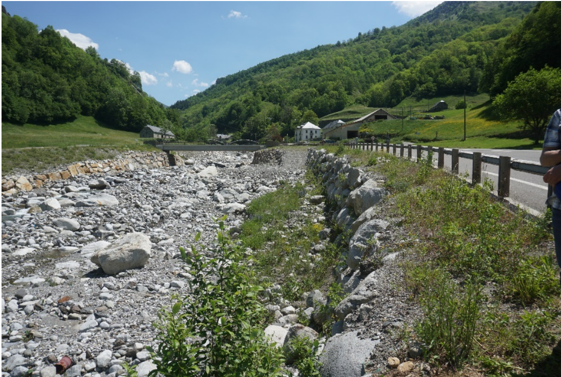
Figure 4.5 Road rebuilt after the 2013 event and sediment transportation into the river
