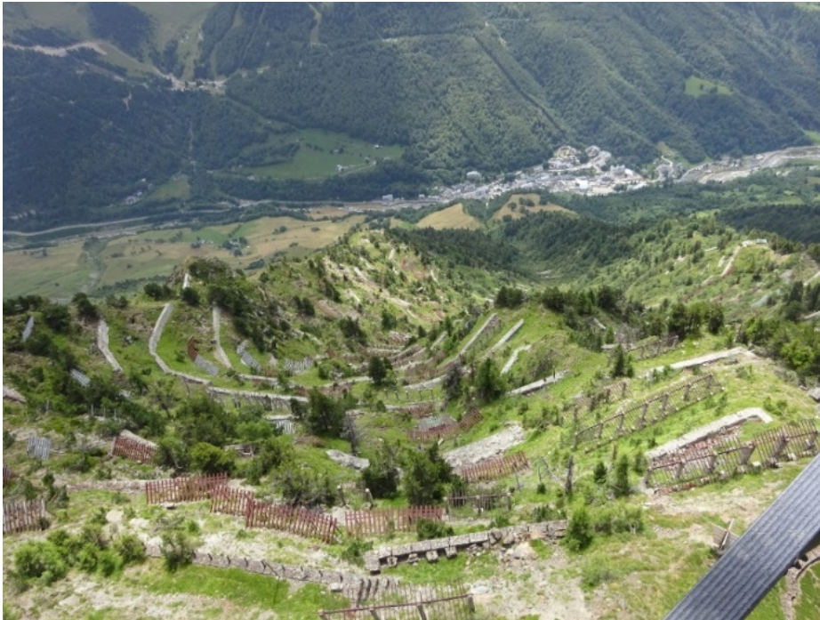
Figure 4.7 Existing protection works in the snow avalanche release area above the village of Barèges.
