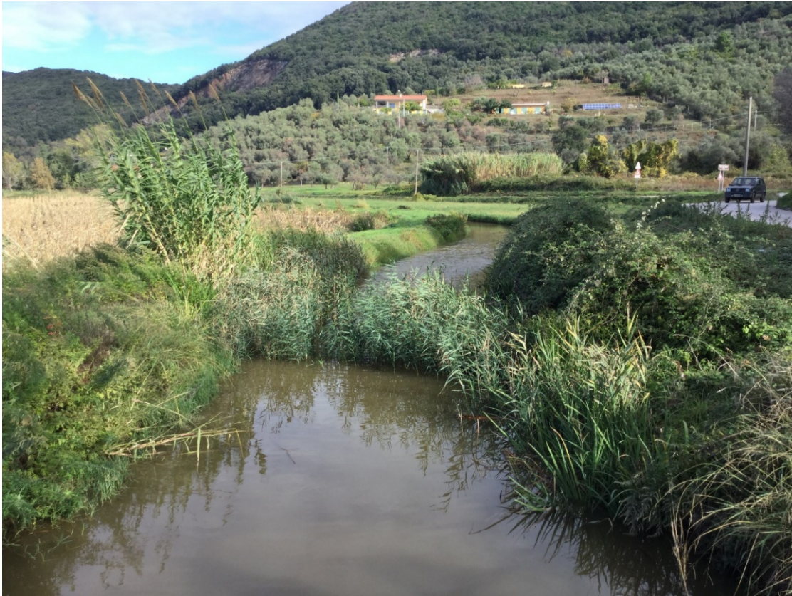
Figure 3.4). The Fossa Nuova channel, seen downstream, which will receive and lead the water from the Serchio River.
