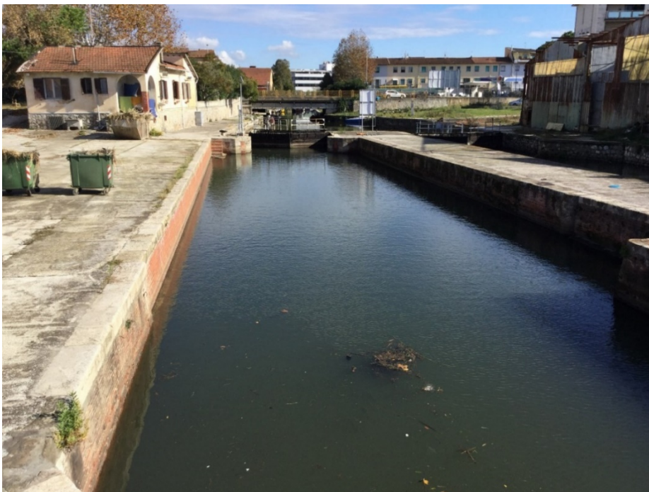
Figure 3.9 (Stop 6). The lock and its upper gate (which is closed) in the channel that connects Lake Massaciucoli to the sea.
