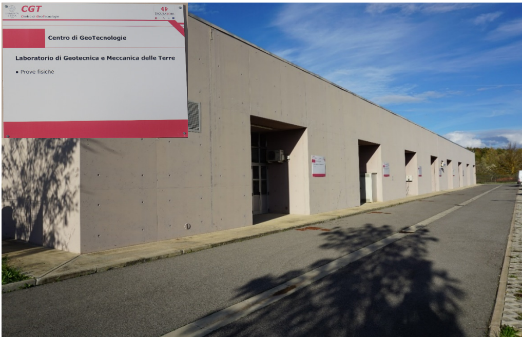
Figure 3.10 CGT's laboratory and warehouse building.
