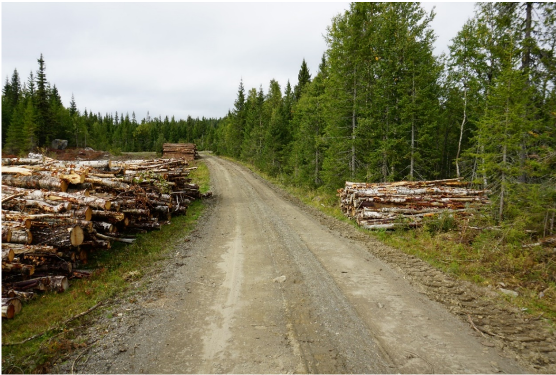
Figure 2.1 One of the bogs to be used is to the right of the road, which will be lifted by roughly 1-2m relative to the lowest point.
