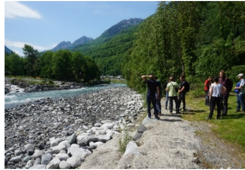
Figure 4.2 Embankment made with stones and cement after the 2013 flood event
