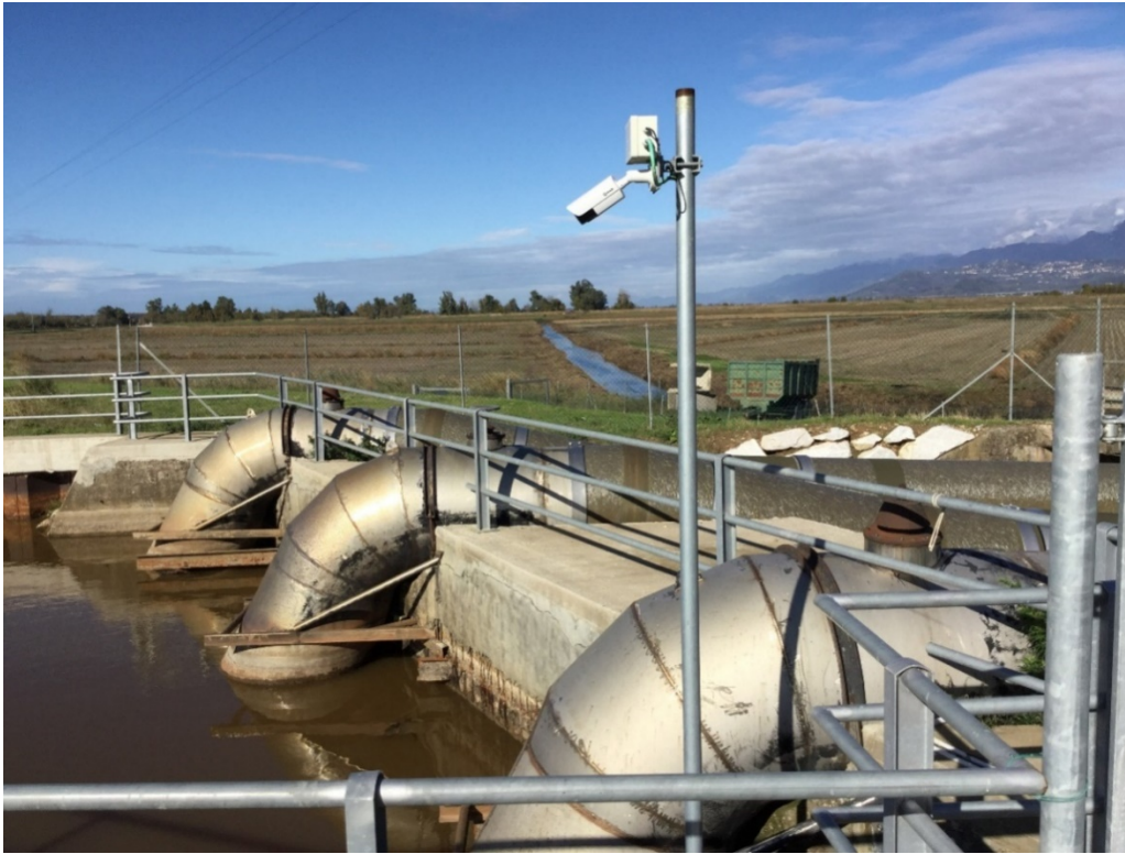
Figure 3.6 (Stop 4). One of the pumping stations. The water in the basin is roughly at sea level, as is the lake level. The lake is right behind the trees in the distance, which mark the levee bordering the lake. The farmland between the pumping station and the lake is roughly 3m below sea level.
