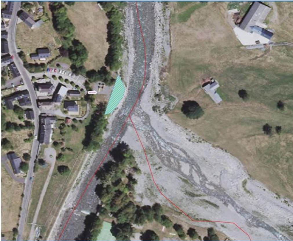
Figure 3.14 The confluence between the Bastan River (from the right) and the Gavernie River. The constructed riverbank to be removed is marked with green shading. Red lines are boundaries between municipalities.
