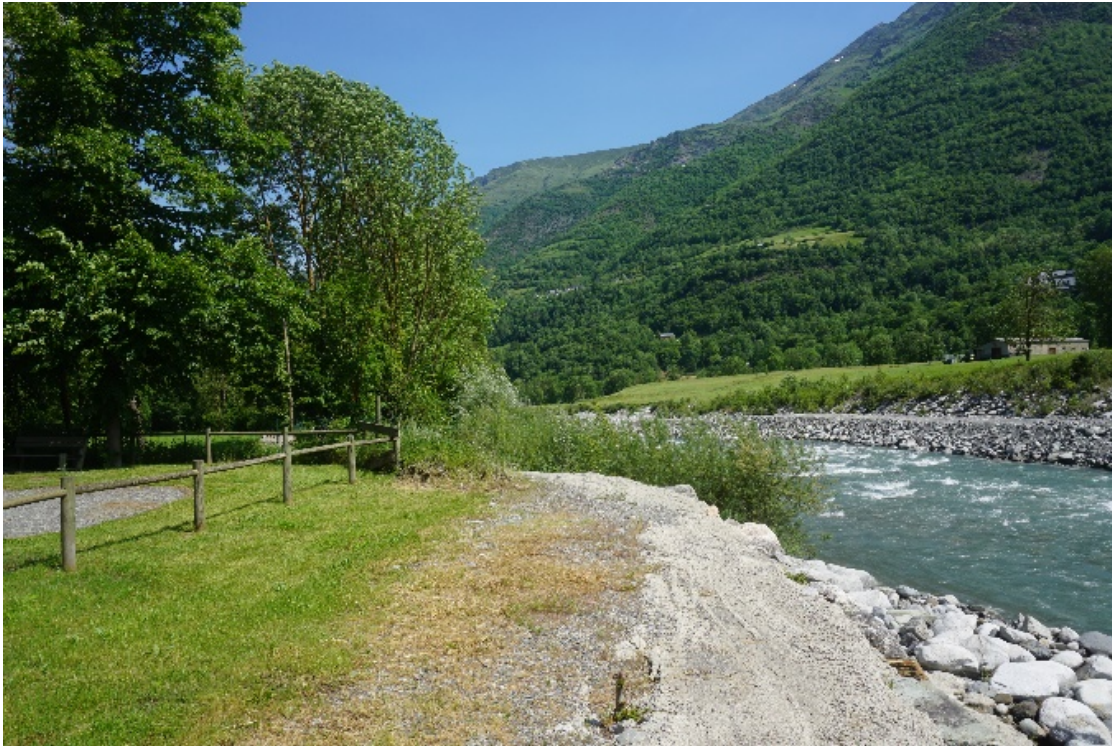
Figure 4.4 Part of the embankment to be removed and renaturalized
