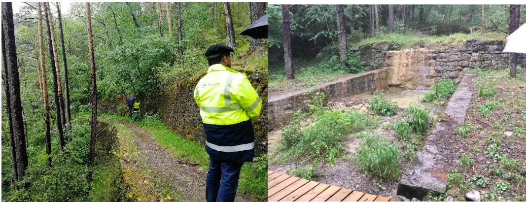
Figure 4.13 Terraces and drainage system, completed in 1905, in Biescas
