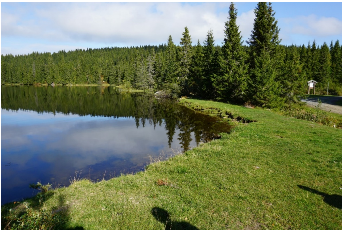
Figure 2.3 Lake Finntjern, with the original dam. The plan is to raise this by 0,5-1,0m.
