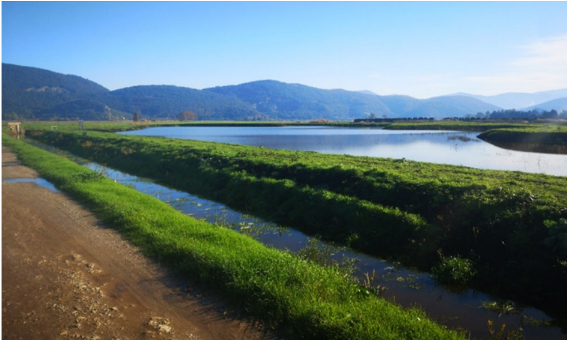
Figure 4-7 The sedimentation basin after completion (Photo: ADBS)
