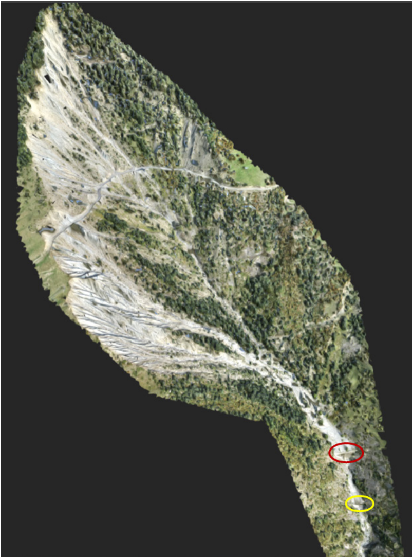
Figure 5-20 Detailed 3D model of the Erill-la-Vall site, before PHUSICOS measures are implemented. The older flexible and fixed barriers can be seen in the red and yellow circles, respectively.
