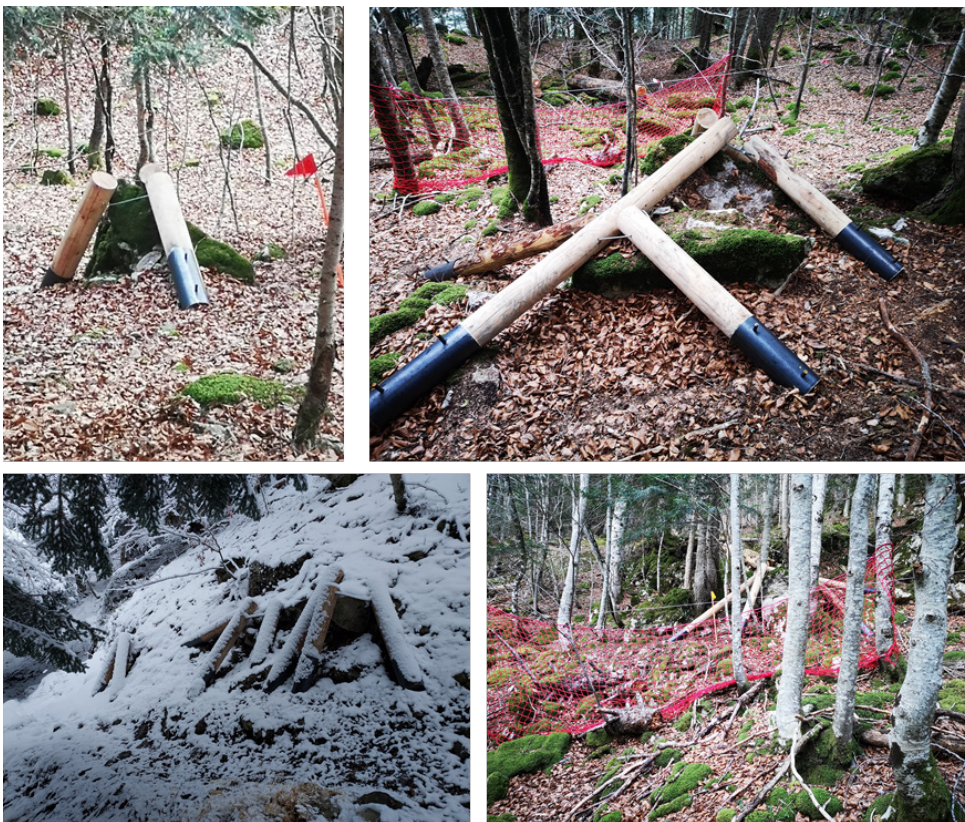
Figure 5-12 Examples of implemented protective structures (based on design principles of Feil! Fant ikke referanse kilden. in the slope at Artouste (Photo: S. Fábregas)
