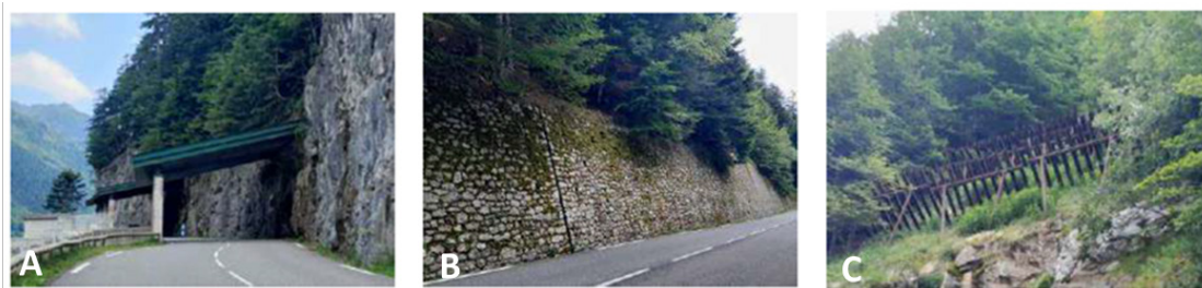
Figure 5-7 Photos of older existing measures. A) Galleries for snow avalanches installed at the confluence of Zone 2 with the road. B) Masonry wall built at the intersection of Zone 4 with the road. C) Avalanche fences that act as shields against falling blocks at the intersect of Zone 3 with the road. (Photos by EGTC Pirineos- Pyrénées)
