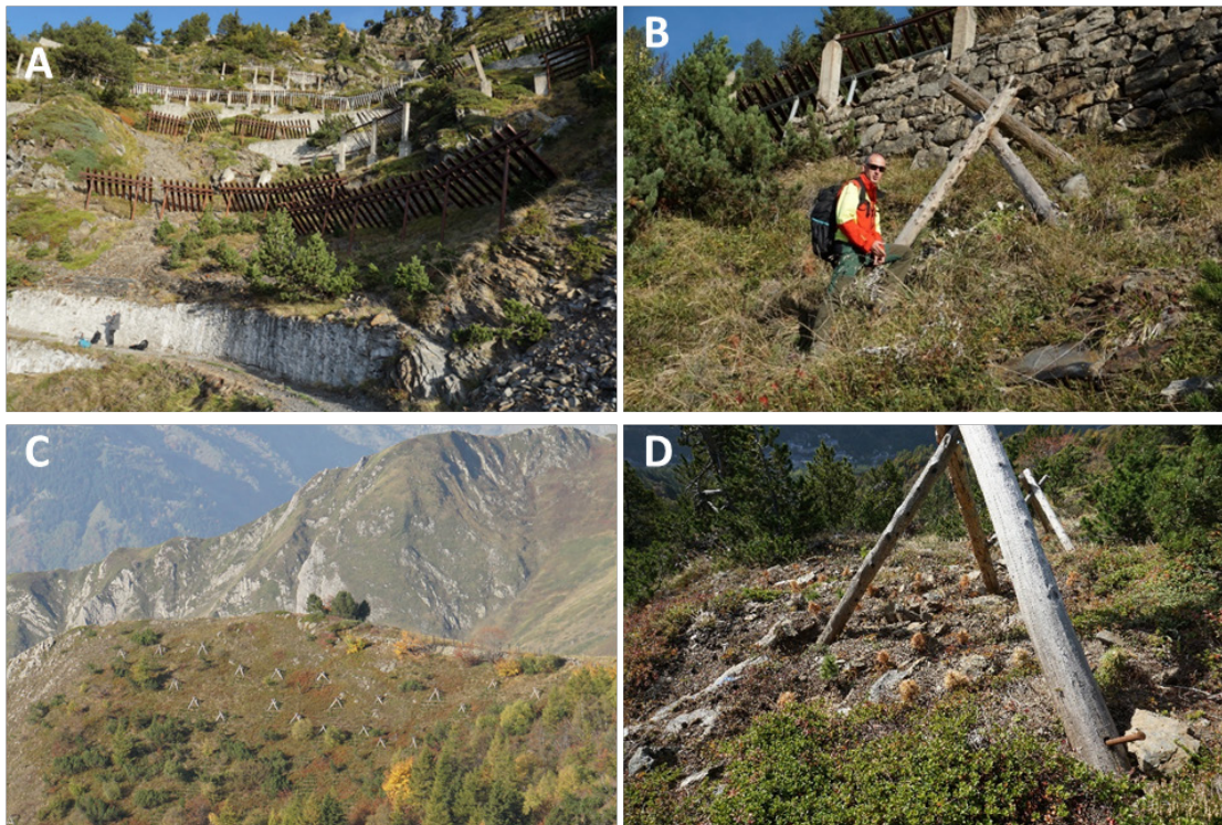
Figure 5-14A) 'Grey' structures in the slope above the access road from the helicopter platform to the construction site for the shelter. B) One of the tripods for protection of new plants. C) Tripods protecting plants in a more barren part of the avalanche release area. Natural forest and old grey structures can be seen in the foreground. D) Example of plant collection where most plants have died, but still enough for the purpose seem to survive.
