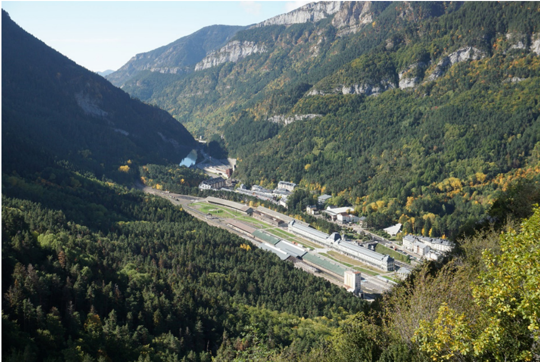
Figure 5-5 The Los Arañones railway station in Canfranc. The forests in the surrounding hill slopes were planted in the beginning of the 20th century.
