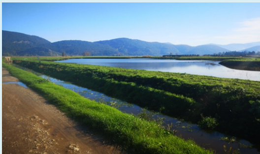
Figure 9: Sedimentation basin after completion (Source: ADBS, 2023).
