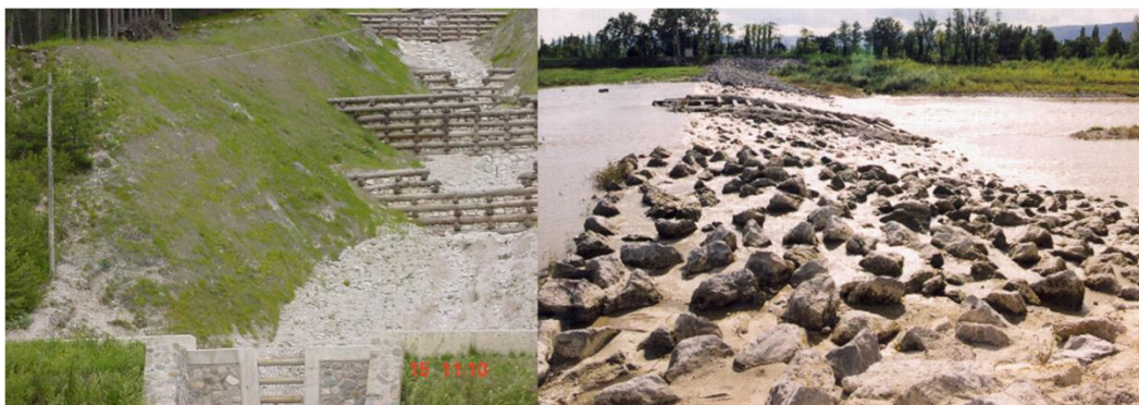
Figure 2-18. Complementary technique. Torrent dams and stone fish ramp (EFIB, Paola Sangalli).
