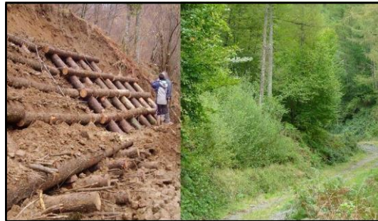
Figure 2-14. Mixed technique. Trellis in Leizaran and after one year (EFIB, Paola Sangalli).
