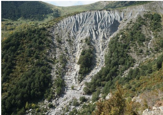
Figure 1-9. Overview on the site of Erill la Vall with the krainer walls and rock terraces at the bottom of the gully.
