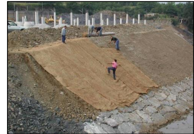
Figure 2-3. Coating technique: placing organic blanket. Valentín Contreras (EFIB, Paola Sangalli).
