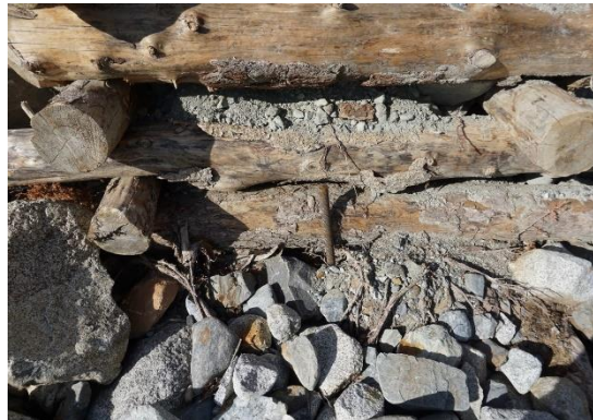
Figure 1-10. Detail on krainer wall filled with material.
