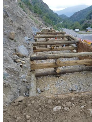
Figure 1-8. Detail on wooden gabions during the construction.
