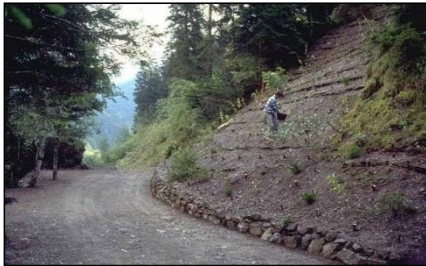
Figure 2-1. Coating technique: broadcast seeding in structure. Florin Florineth (EFIB, Paola Sangalli).
