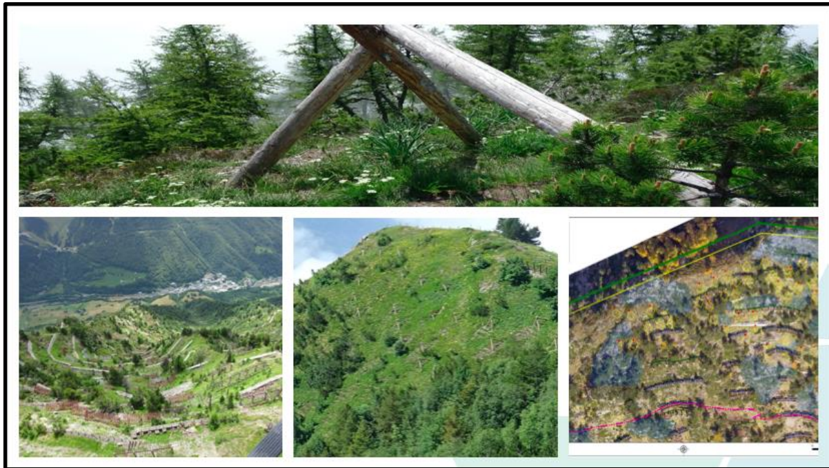
Figure 3-3. Illustrations of the Capet Forest site and NBS implemented by PHUSICOS (wooden tripods and afforestation). At the bottom left of the figure, grey infrastructure can be seen on the slope with the village of Barèges at the bottom.
